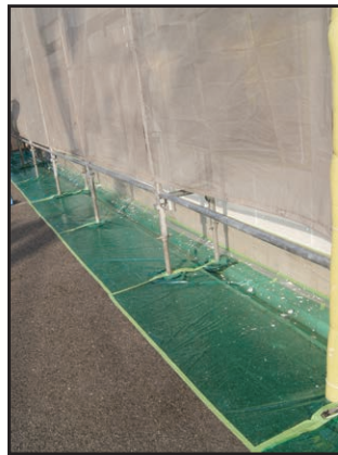
壁側の床面養生に
